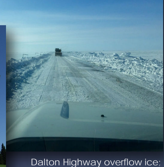
Dalton Highway overflow ice. Photo courtesy of Alaska DOT&PF
