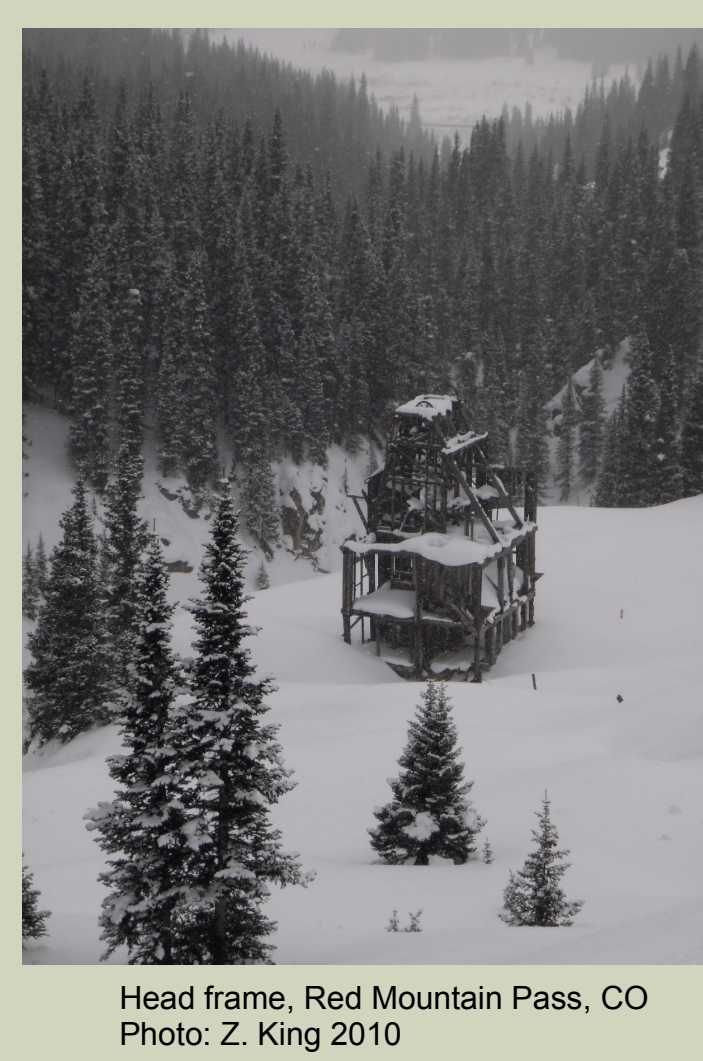
Head frame, Red Mountain Pass, CO Photo: Z. King 2010
