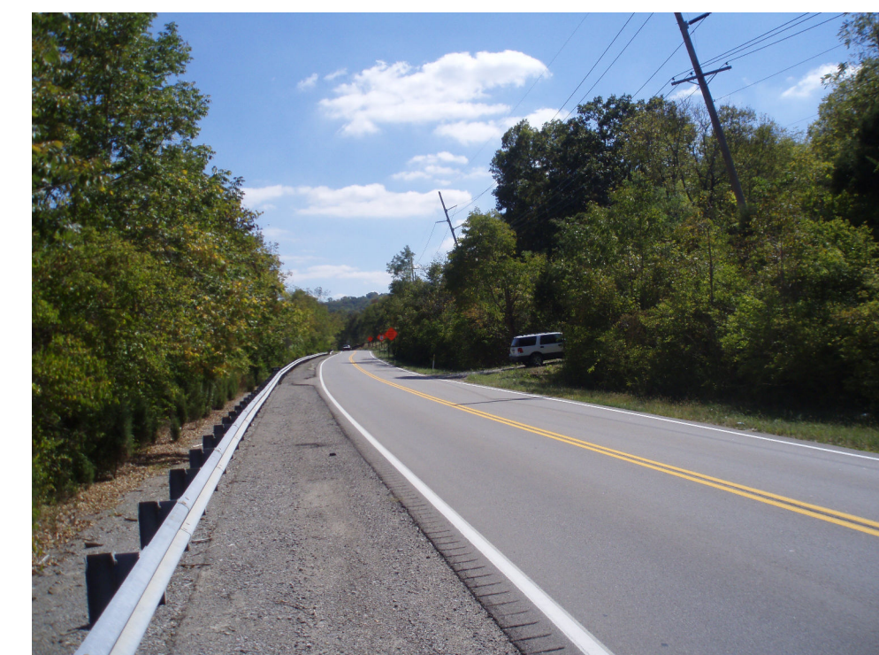
KY 8: Leaning telephone poles on large slide above and below road
