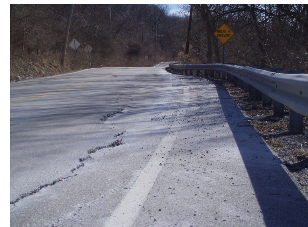
Licking Pike: Scarp and cracks in pavement, slide above and below road
