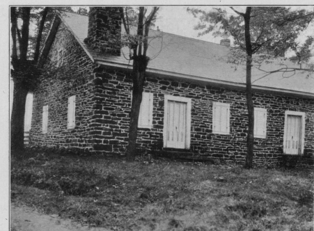
PLATE 20.—OLD QUAKER MEETINGHOUSE NEAR BERMUDEAN CHURCH Built in eighteenth century of Triassic red sandstone
