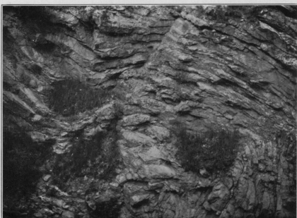
PLATE 15.—FOLDED THIN-BEDDED WEVERTON QUARTZITE AT EAST PORTAL OF WESTERN MARYLAND RAILWAY TUNNEL IN TUNNEL HILL
