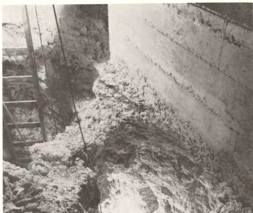
A. Cavity in limestone under new Navy Hospital, showing detail of footing.
