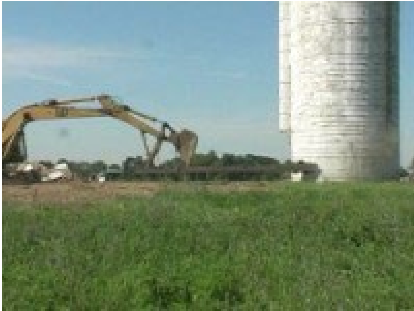
100 Year Old Silo Demolished YouTube - https://www.youtube.com/watch?v=nksEVPQ6cvs
