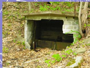
Figure 10. Mine water discharges from a trough built into an opening in the Ames Mine in the New River Gorge east of Fayetteville, WV. (photo by G.H. McColloch)
