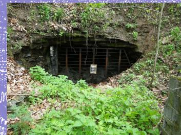
Figure 12. An opening in the Dubree No. 4 mine in the Sewell coal near the site of Nuttallburg in the New River Gorge near Fayetteville, WV, has no water emerging from it. The grate over the mine opening provides access for bats.
