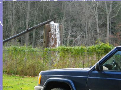
Figure 1. Water discharging from a powerhole in the down-dip end of the Summerlee mine in the Sewell coal seam emerges from a pipe at Dempsey, WV, where the water is treated. The mine is approximately 340 feet below the surface at this location. (photo by G.H. McColloch)
