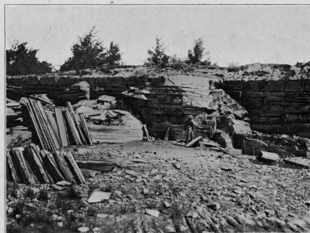
FIG. 6.—FLAGSTONE QUARRY AT HEAD OF CORY CREEK, EAST OF MANSFIELD.
