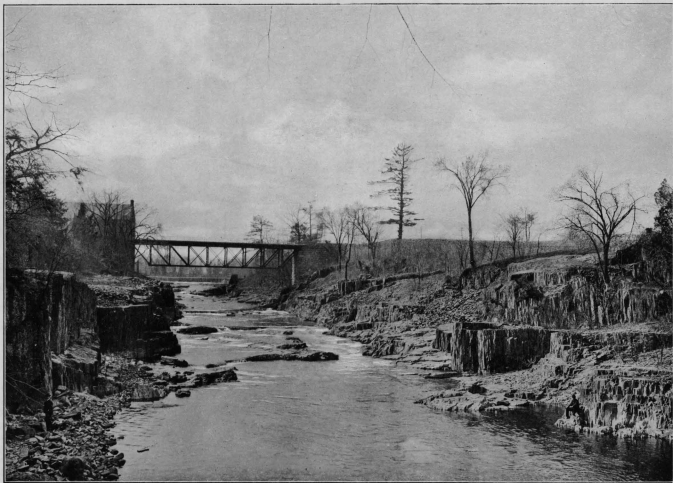
FIG. 21.—LITTLE FALLS OF PASSAIC RIVER, AT THE TOWN OF LITTLE FALLS, N. J.
