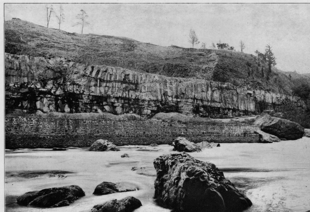
FIG. 16.—CONFORMABLE CONTACT OF BASALT OF THE FIRST WATCHUNG FLOW ON NEWARK SANDSTONES, BELOW FALLS OF THE PASSAIC, PATERSON, N. J. The sandstone forms the base of the section immediately above the retaining wall and is overlain by massive-bedded lava, with finely columnar basalt on top.
