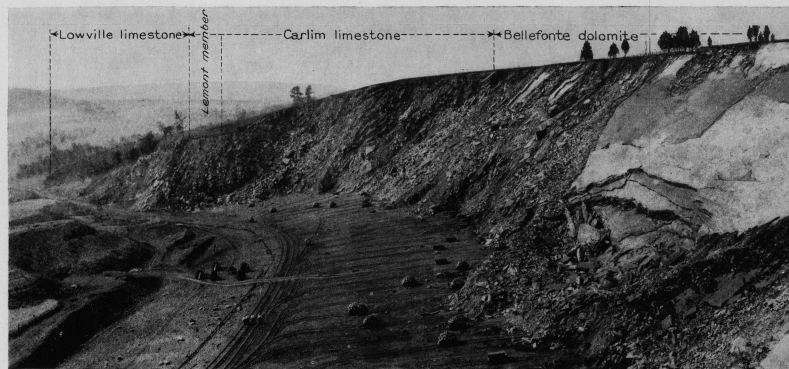
PLATE 25.—VIEW OF CLOVER CREEK QUARRY AT SPARR Mainly in Carlim limestone. Beekmantown dolomite at bottom. Looking southwest.
