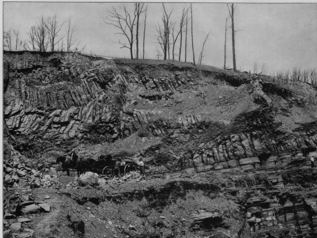
FIG. 27.—QUARRY NEAR UPPER MONTCLAIR, N. J., LOOKING NORTHWEST. Watchung basalt lying conformably on Newark sandstone. The sandstone is both bedded and jointed; the basalt is irregularly jointed and columnar.
